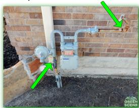
• The corrugated stainless steel tubing (CSST) gas supply line bonding/grounding wire was not observed or not bonded correctly. This wire should be a #8 AWG wire. This condition should be further evaluated by a licensed electrician.
