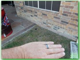
• Fill dirt is needed on the west side of the structure. The low spots in the finished grade (ground) adjacent to the foundation perimeter wall need to be filled in to help prevent water from standing and/or ponding next to the foundation area.
