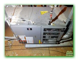
• The heater gas supply line is not equipped with a sediment trap just before the gas appliance connector. This condition does not meet current installation requirements and should be corrected.
